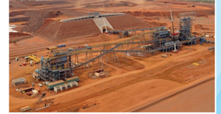
Fortescue's Chichester Hub consists of Christmas Creek and Cloudbreak iron ore mines
